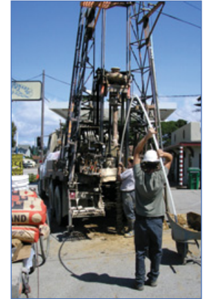
A gas station site in Watsonville, California. Five 3-Channel CMT Systems were installed to monitor gasoline contamination and MTBE plume. Installations were completed within hollow stem augers using bentonite and sand layers to isolate each monitoring zone.
